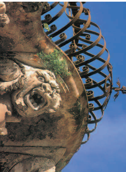
A typical Baroque balcony
